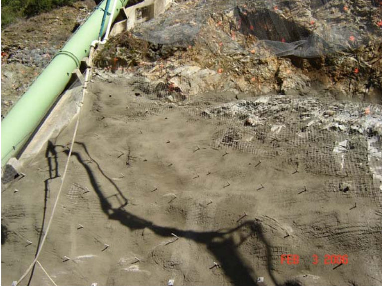
Placing the shotcrete over the mesh and soil nails.
