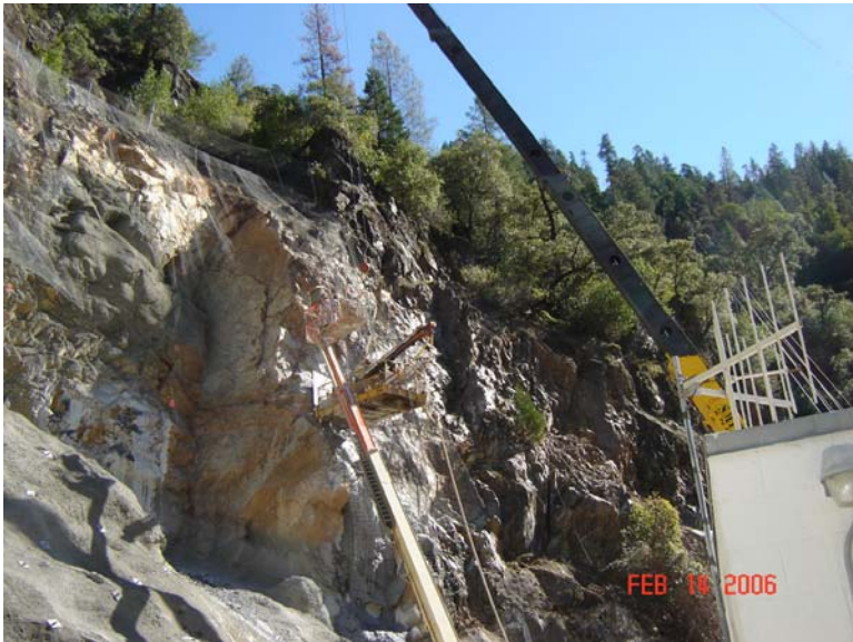
Drilling the rock bolts from the basket drill.
