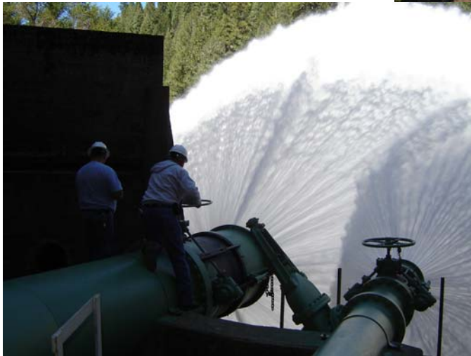
Photo above – Toe of Little Grass Valley Dam with Howell-Bunger valve fully opened.
