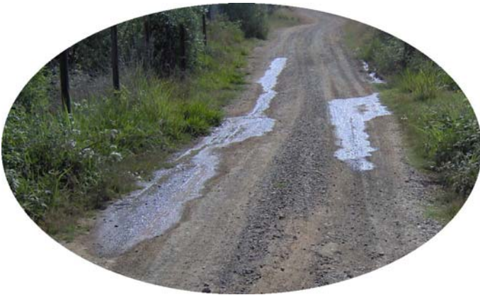
The photo above shows the currently leaking water line that has previously been fixed numerous times.
