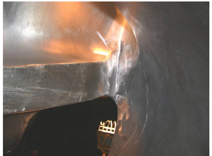
Photo 6: Final weld repair after polishing
