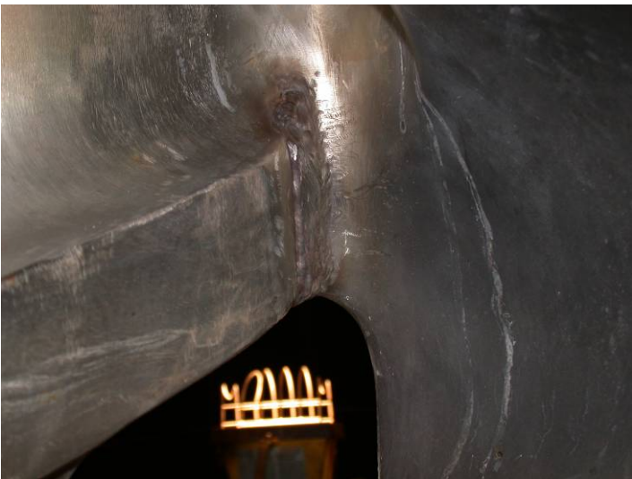
Photo 5: Final weld before grinding
