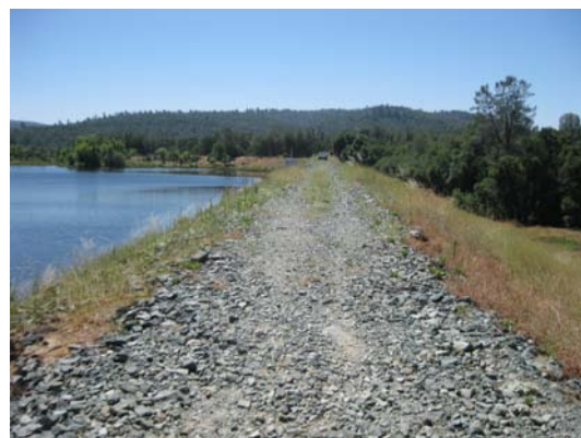
Miners Ranch Dam Crest
