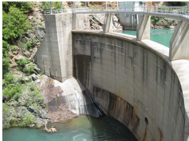
Forbestown Diversion Dam
