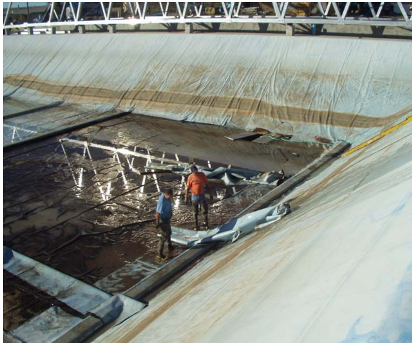
Figure 1. Careful removal of blue hypolon while not damaging the remaining black bottom liner
